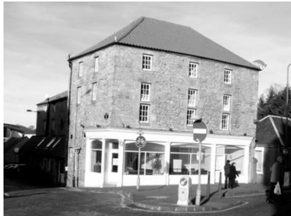
The much-altered mill – but still recognisably the same building as in old drawings
