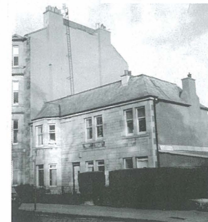
84-86 East Claremont Street
