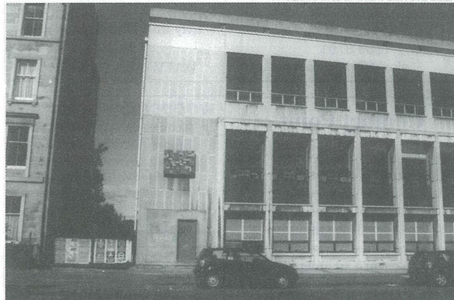
The telephone exchange in East London Street. Not a pretty sight; but could the facade be softened, and the wider pavement in front of it be used for greenery?
