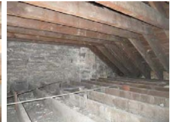
Roof structure at north wing
