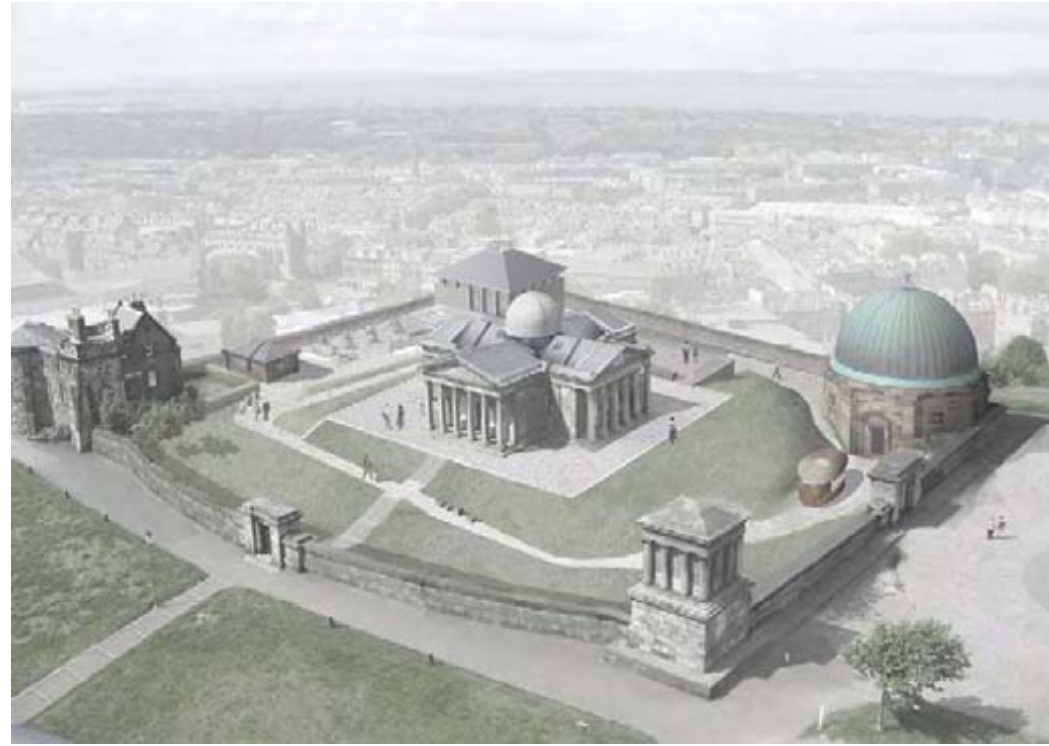
Site aerial (as viewed from Nelson Monument) indicating scale and roof form of new north-west pavilion in the context of the Coty Observatory compound.
