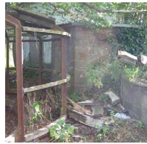
Aerial building and dome frame
