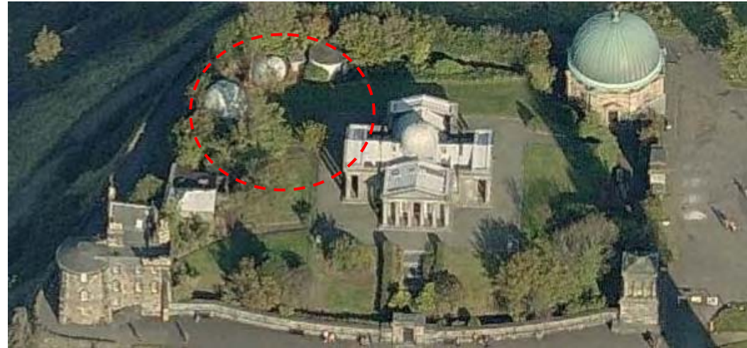
Structures to be removed are focused to the north-west corner of the site
