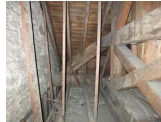
Roof truss at Dome
