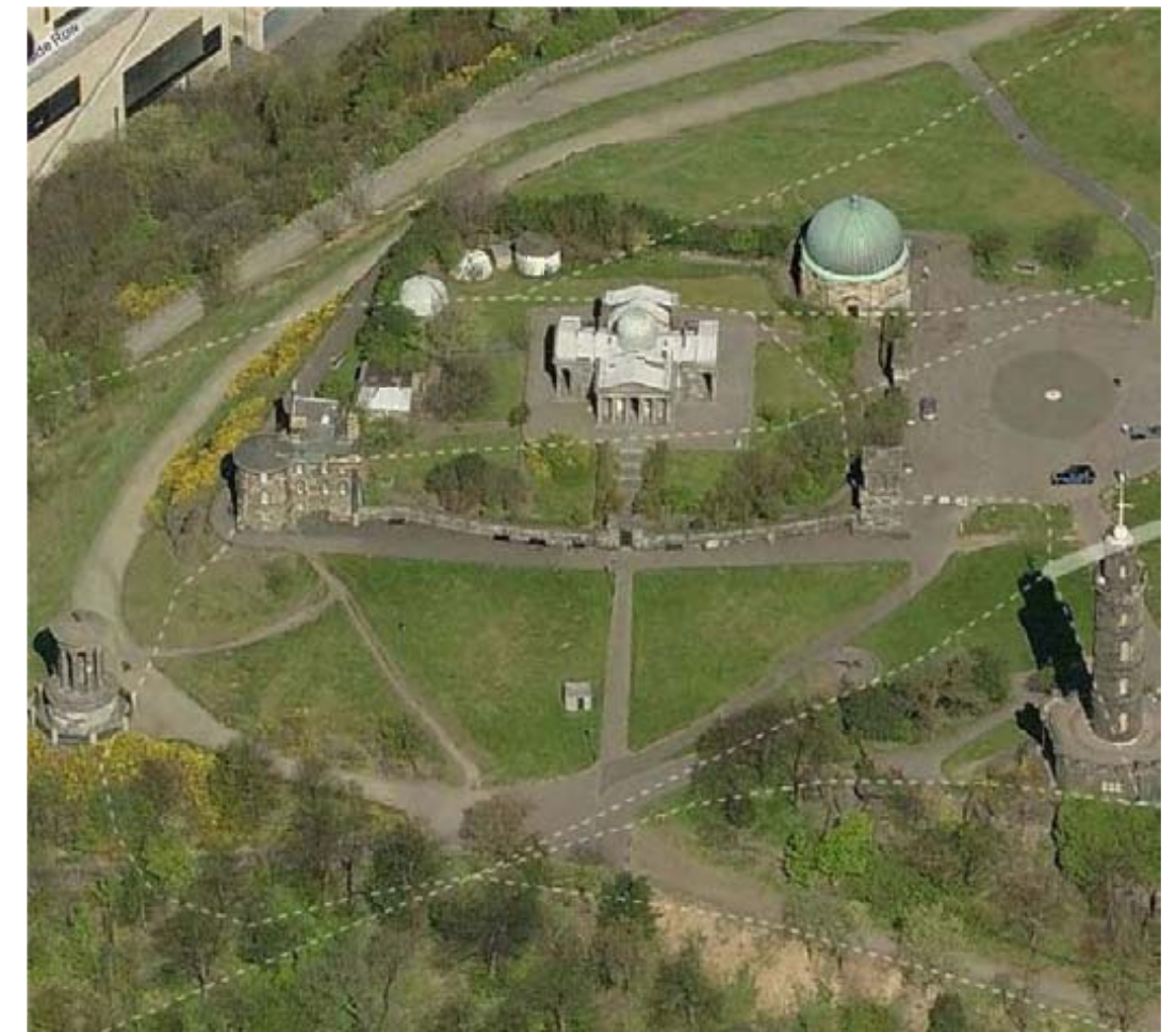
City Observatory Complex: building elements
