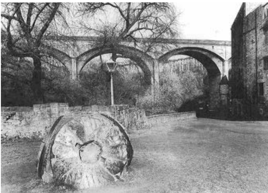
Eric le Mare, Miller Row and Dean bridge 1960s (RCAHMS)
