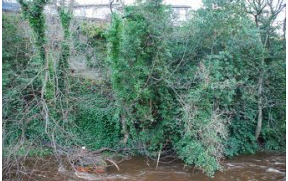
Riverbank at Upper Dean Terrace
