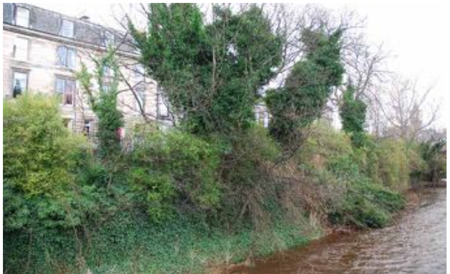
Riverbank at Upper Dean Terrace
