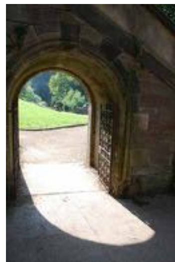
Accessible entry to Walkway at St Bernard's bridge from Saunders Street
