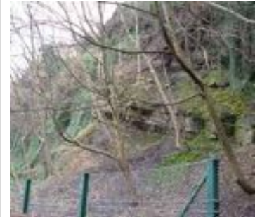
Mudstone exposure underneath the Dean Bridge (CEC)
