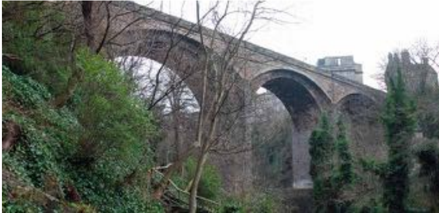
Dean bridge from Belgrave Crescent Gardens
