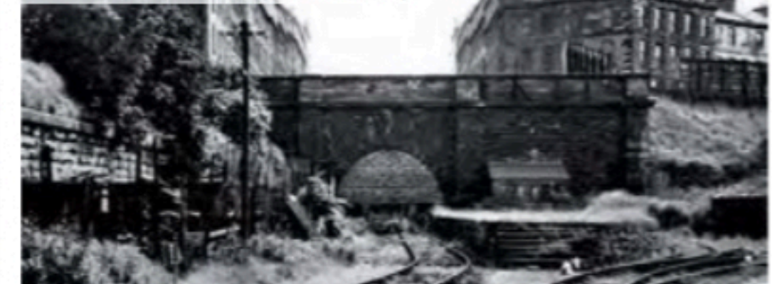
SCOTLAND STREET RAILWAY (LOOKING SOUTH)
