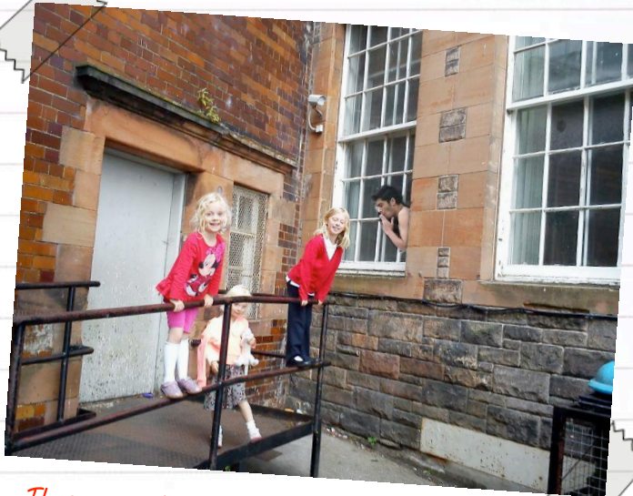
These are the windows of Unit 19. The man in the window has been Photoshopped into the picture for illustration purposes
