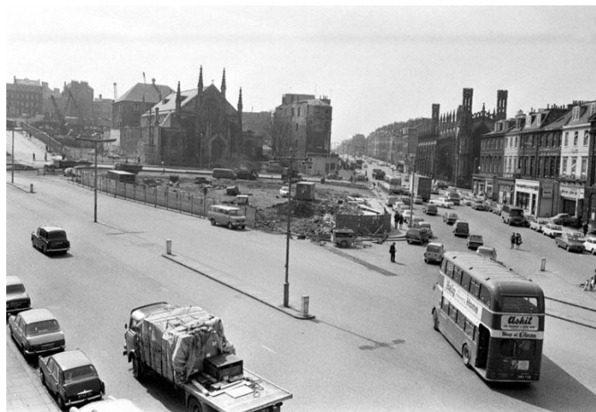
Figure 3 - Photograph of the site – early 1970's
