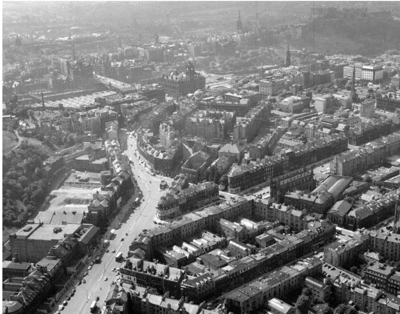
Figure 5 - Aerial view taken in the 1950's
