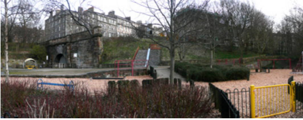
FIG 28 Present condition of adventure playground and area adjacent to tunnelmouth viewed from cycle path.
