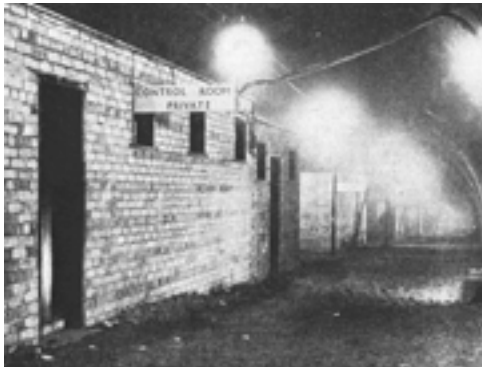
FIG 13 LNER WWII emergency control centre. [Evening Dispatch 16/03/1945]
