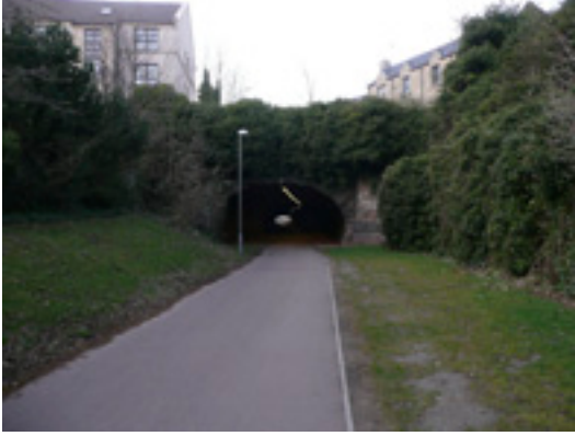
FIG 26 View into the recently opened Rodney Street Tunnel cycle path
