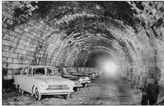
FIG 14 Cochrane's Garages used the tunnel for car storage
