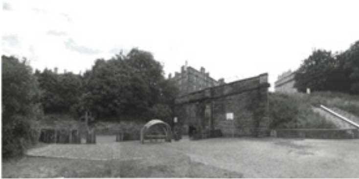
Scotland Yard Playground prior to implementation of phase 1 enabling works.
