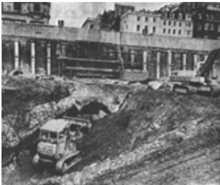
FIG 15 (left) Southern end of the tunnel demolished during excavations for the Princes Mall foundations. [Edinburgh Evening News 05/01/1983]
